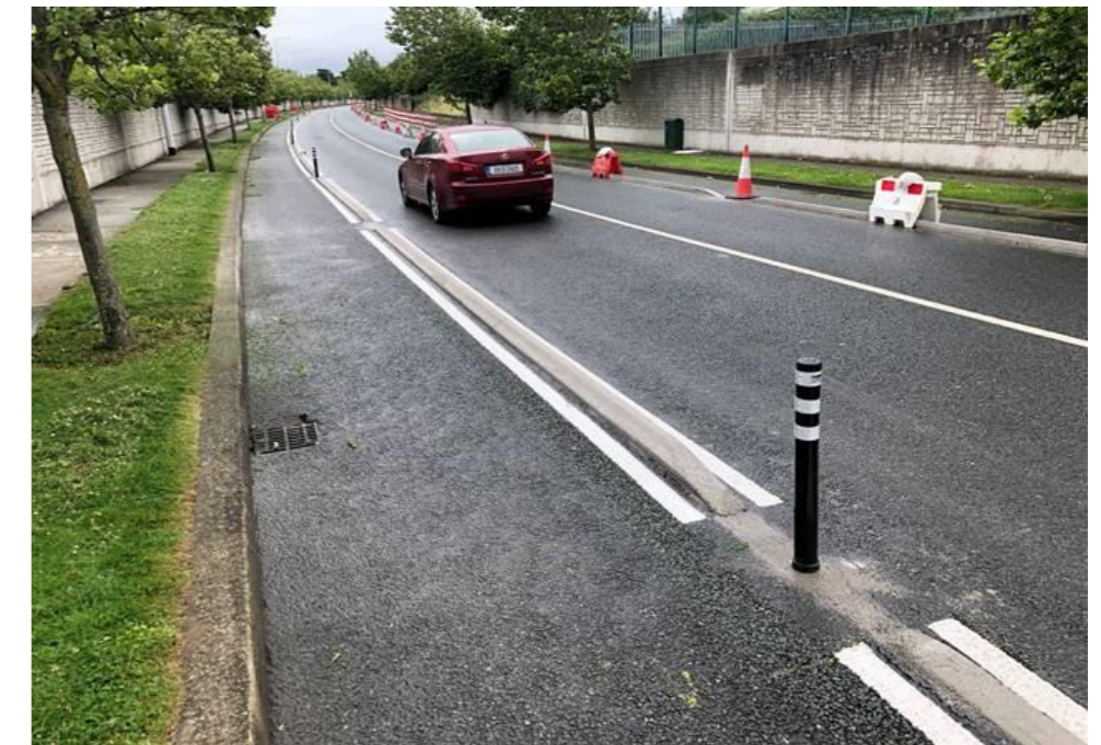
Figure 9: Retro-fit kerb solution (example shown is Benildus Avenue)
